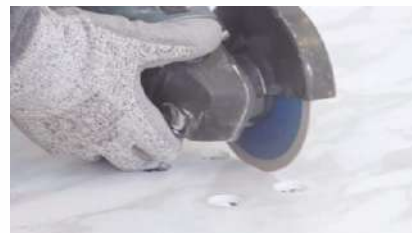
2. Cut with Diamond Blade Angle Grinder
