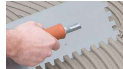
1. Cement laying on Floor
