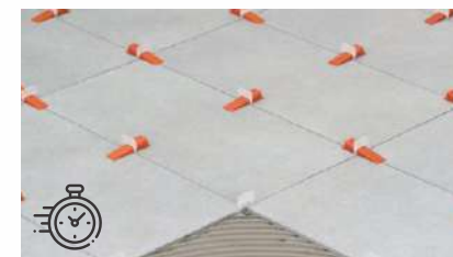
5. After Levelling Process leave it for 8-10 hrs.
