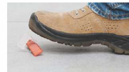
6. Remove Wedges ones it Dry
