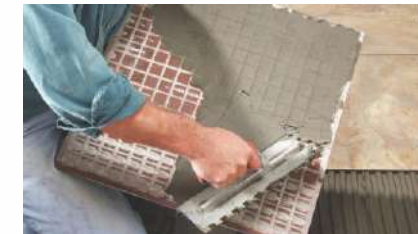
2. Cement laying on Tile
