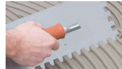
1. Cement laying on Floor
