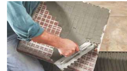
2. Cement laying on Tile
