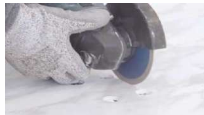
2. Cut with Diamond Blade Angle Grinder
