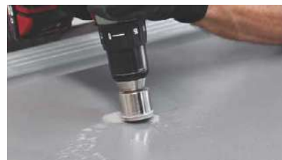
1. Round Cut with Diamond Blade Drill
